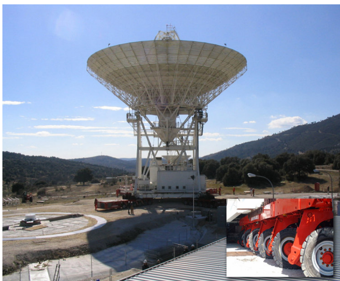
Giant Deep Space Network antenna in Madrid is moved using four 12-axle, 24-wheel crawlers.
