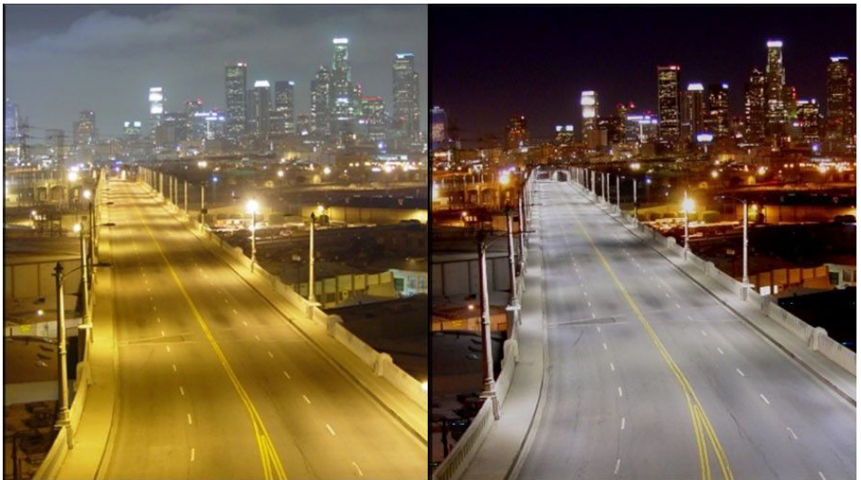
Before and after pictures of replacement lighting at the 6th Street Bridge over the Los Angeles River. The second picture shows improvements in some aspects of light pollution, as light is not directed to the sides and upwards from the upgraded fixtures, reducing skyglow. However, it also shows the use of brighter, whiter LEDs, which is not generally ideal, along with increased light bounce back from the road. Credit: City of Los Angeles
